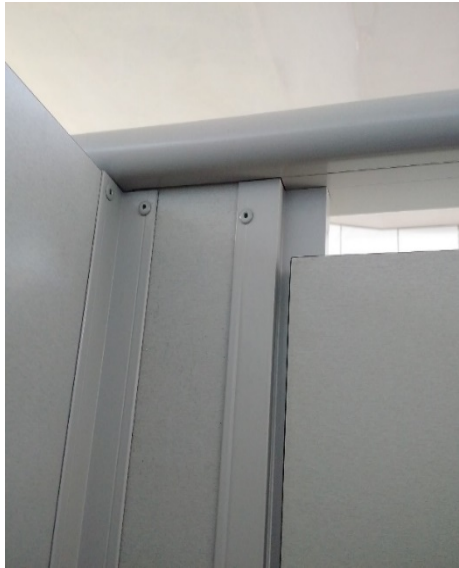
Headrail and pilaster join from inside the cubicle
